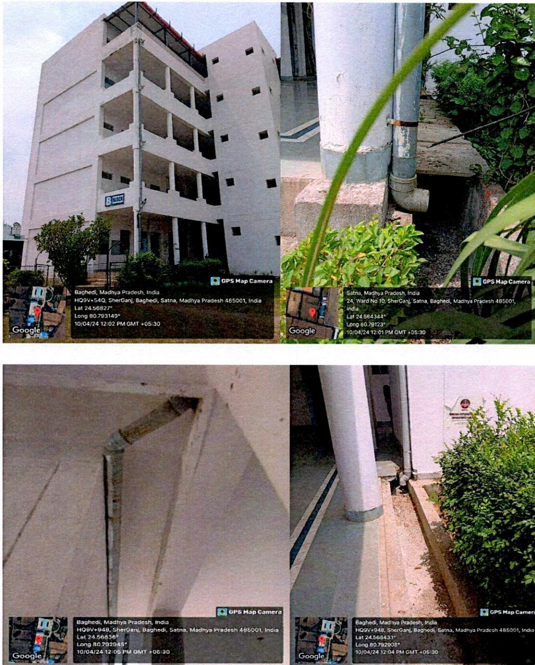
Figure 3: Rain water harvesting (B Block)
