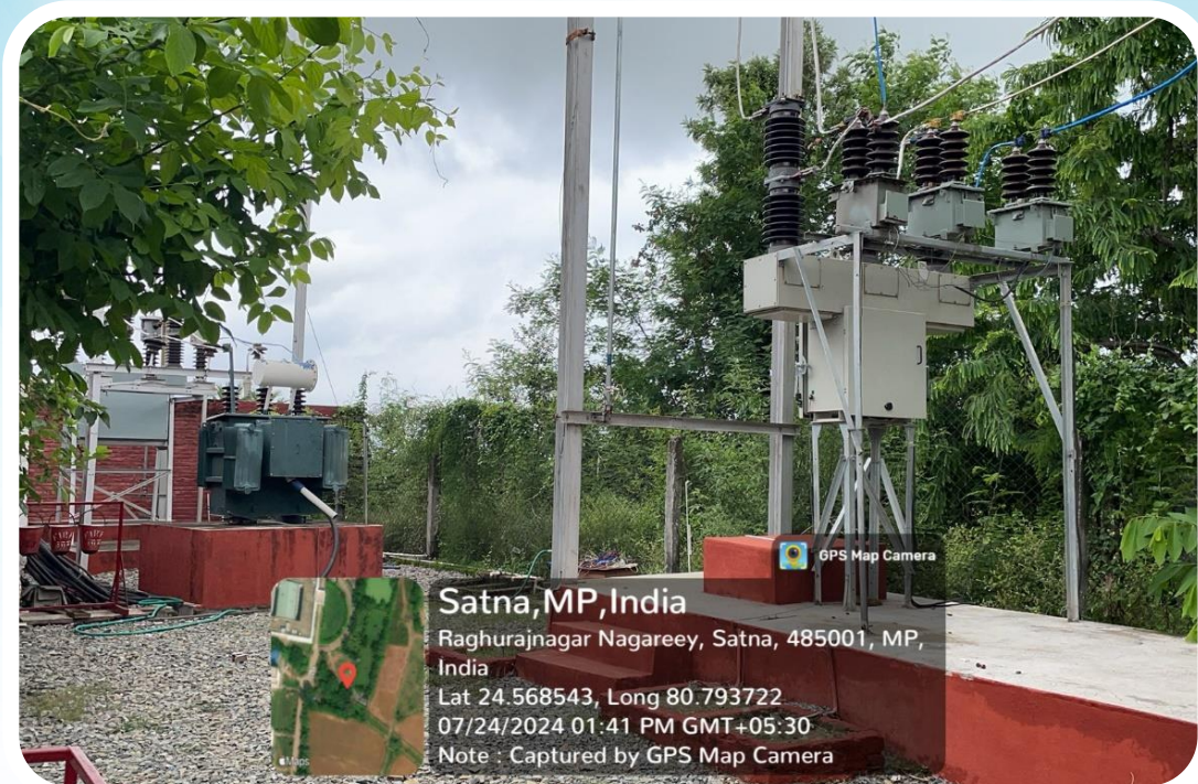
Photo 13: Wheeling the grid
