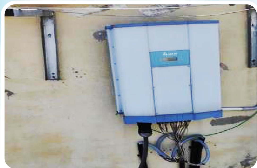
Photo 8: Wheeling the grid
