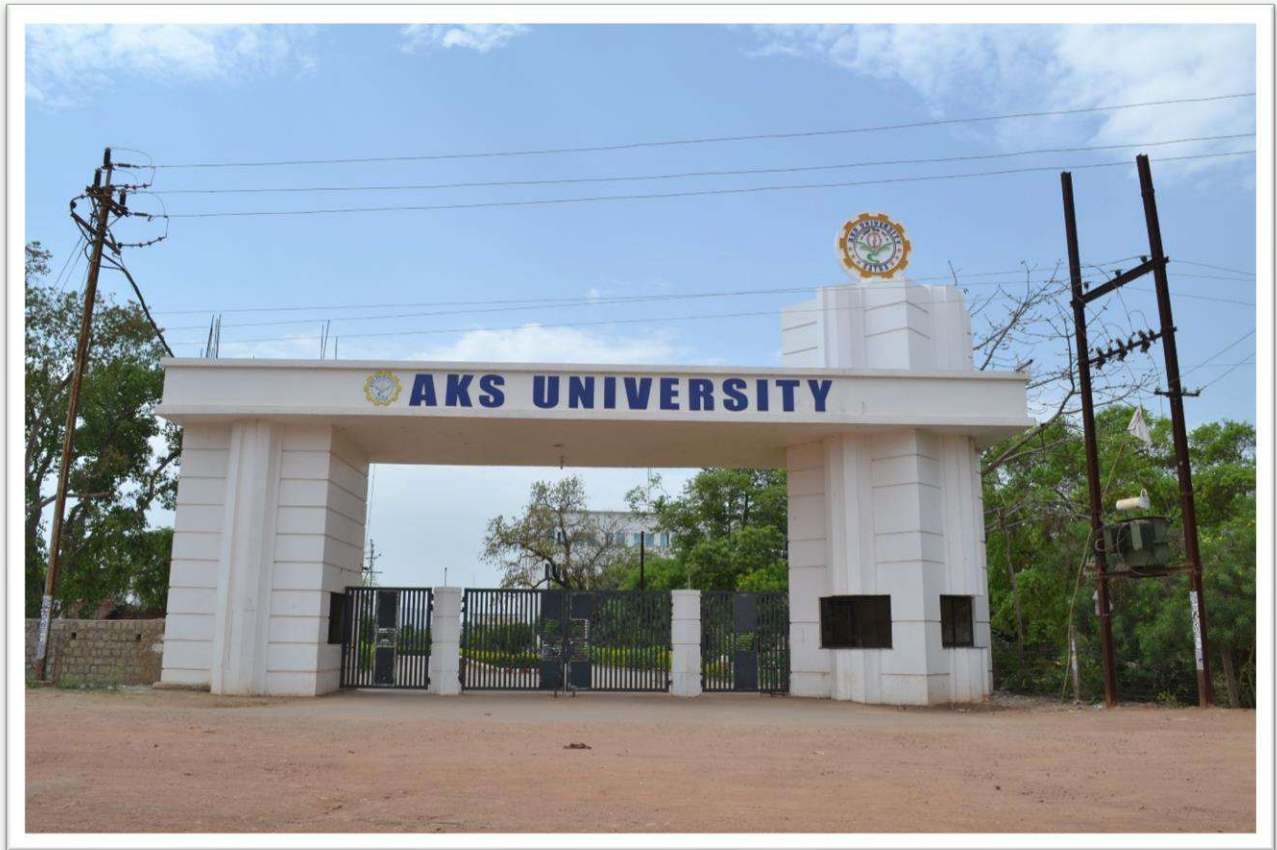
MAIN ENTRANCE GATE
